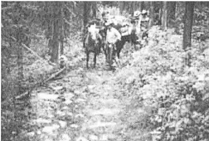
*Figure 9—Standing water results in soft, boggy tread. The very best drainage designs are those built into new construction. These include frequent grade reversals and outsloping the entire tread. The classic mark of good drainage is that it's self-maintaining, requiring minimal care.*
