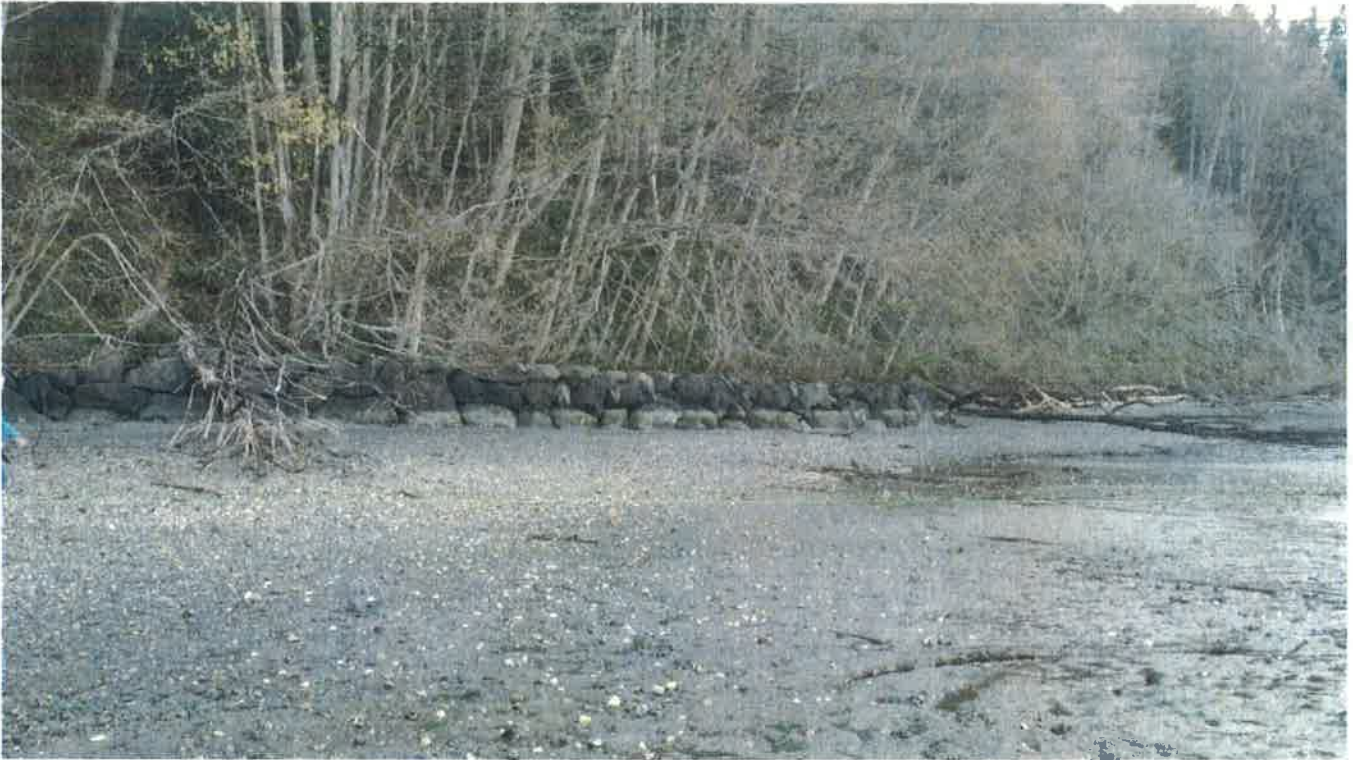
Shoreline armoring impeding natural beach processes.
