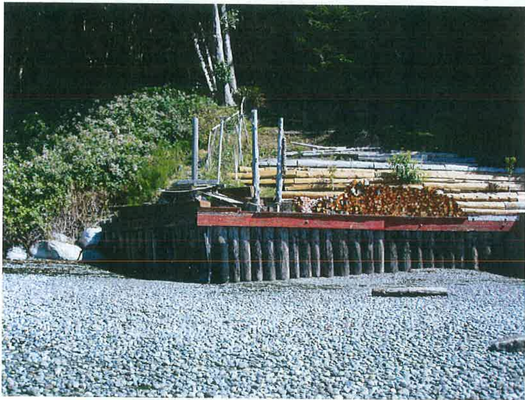
Creosote bulkhead sticking out into the intertidal
