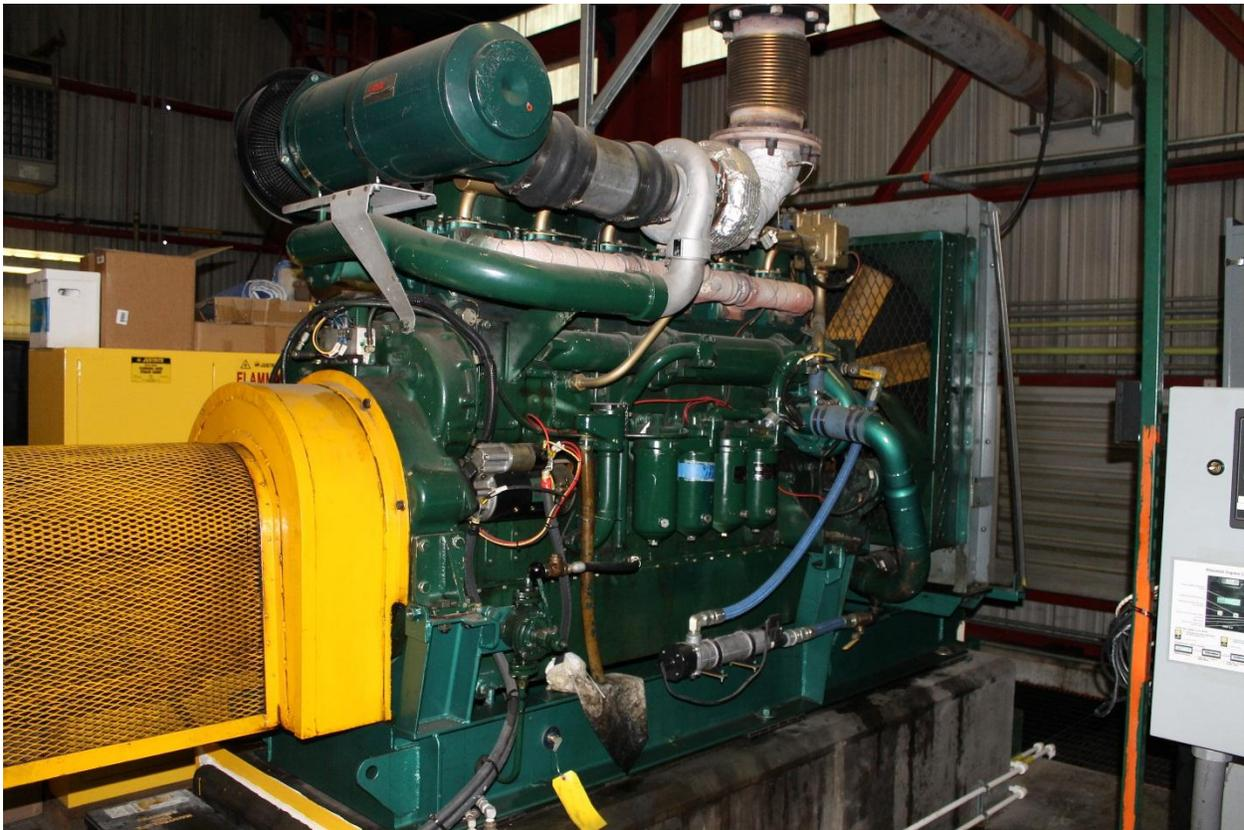
**Figure 5-1 Mitsubishi Model S6N-PT Turbocharged Diesel Engine for Pump P2**
