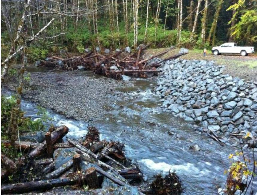
Figure 3: Looking U/S from bridge at Bank Roughening Jam, Willoughby Creek, WA.
