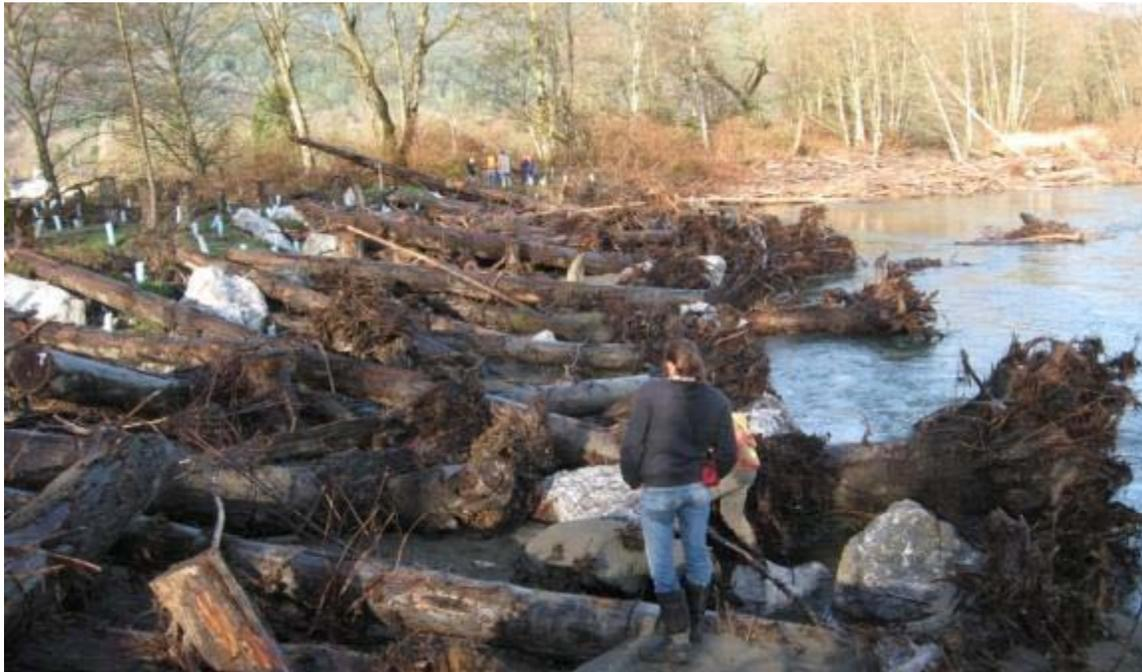
Figure 2: View looking downstream along the Bank Roughening Jam that was installed in 2009, South Fork Nooksack River near Acme (February 4, 2010).
