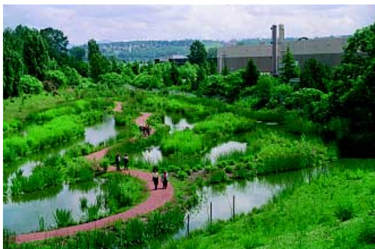
The parklike Waterworks Garden at the East Treatment Plant treats stormwater while providing open space for wildlife and people.
