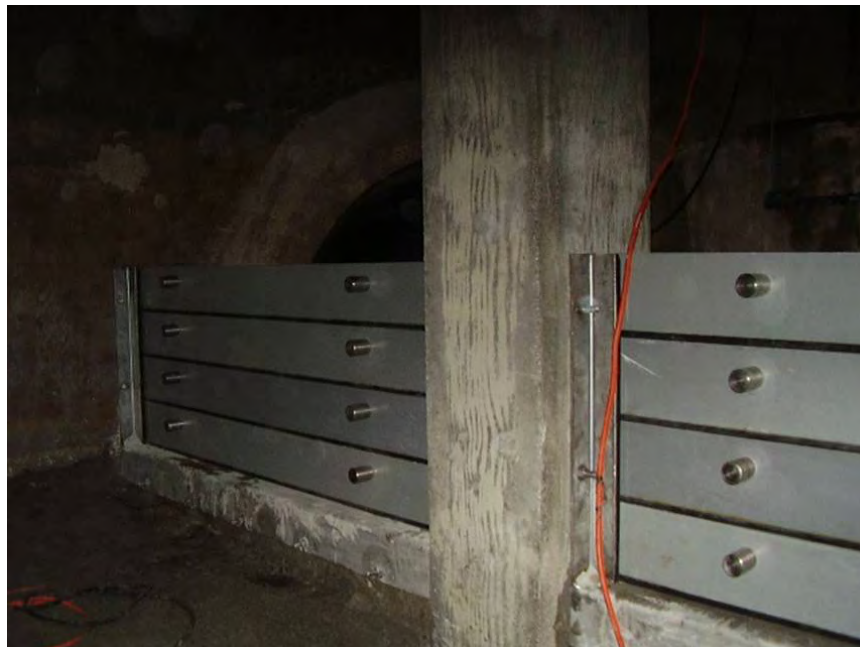
Figure 2. Stoplog Installation at Valley Connection from East Lake Union
