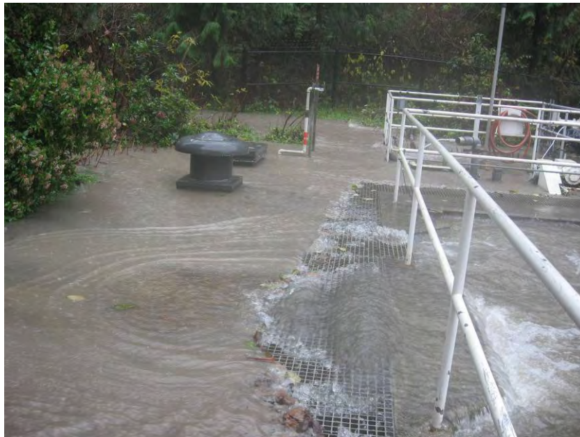
Figure 4. Pipers Creek Overflowing into Carkeek CSO Plant on December 3, 2007.
