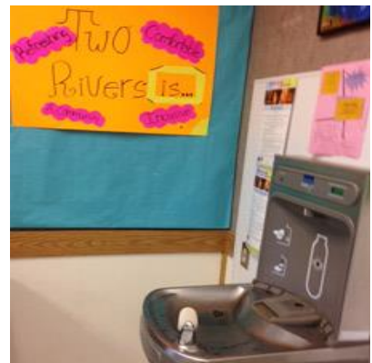
Water bottle refilling station to encourage students and staff to use reusable water bottles
