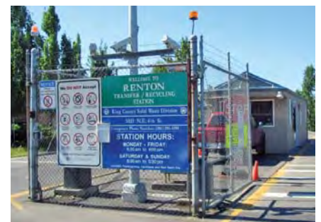
Main entrance and scalehouse
