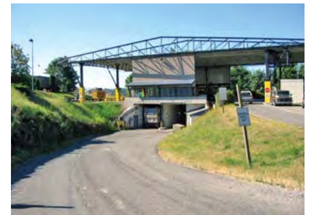
Transfer building: upper left side for commercial customers, lower center for trailers, and upper right for self-haul customers
