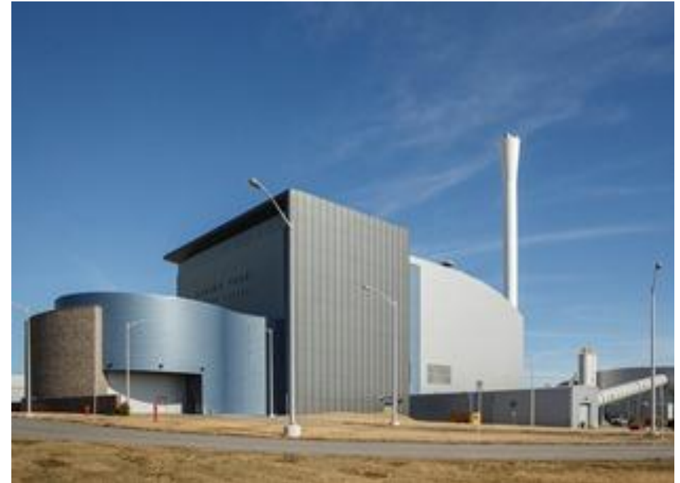
Durham/York WTE facility in Ontario
