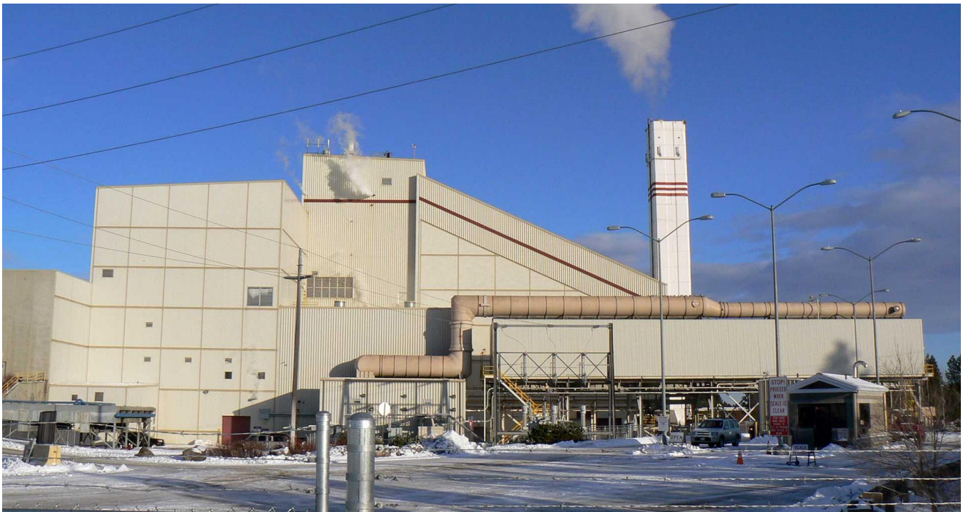
Figure 2-2: Waste-to-Energy (Mass Burn) Facility – Spokane WtE Facility, Spokane Washington
