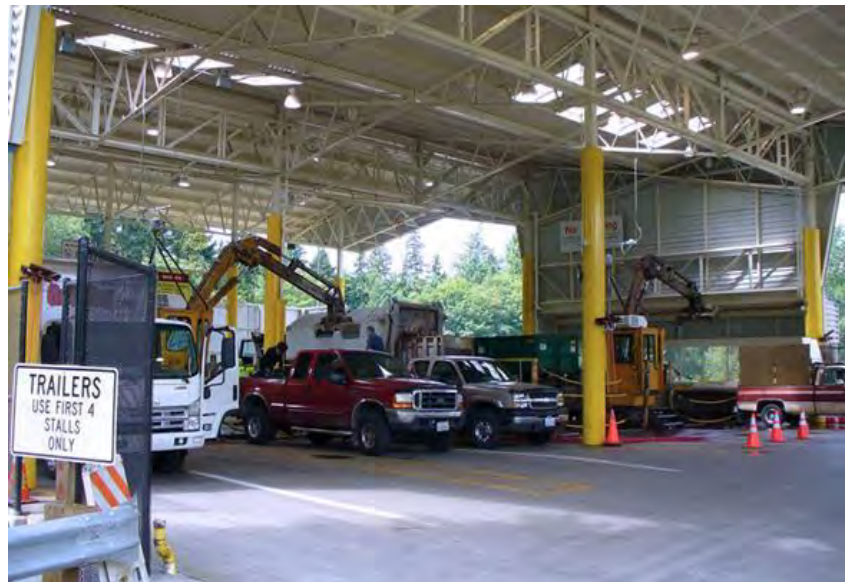
Interior of current Houghton Transfer Station.
