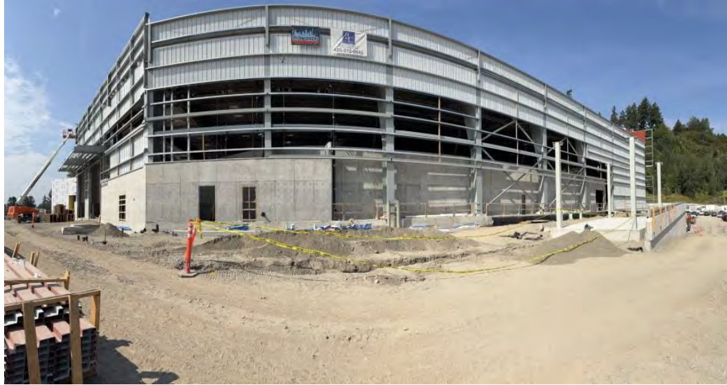
Construction continues on the South County Recycling and Transfer Station project.
