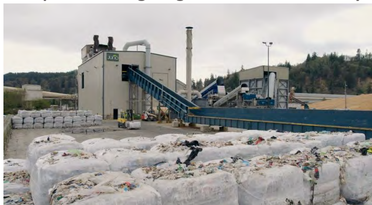
The Juno mixed waste processing facility.
