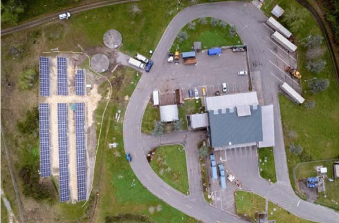
The Solid Waste Division worked with local installer Western Solar to build the new array – a connected network of 348 solar panels – on previously unused land next to the Vashon transfer station.
