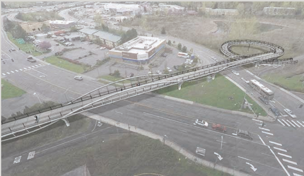
The new pedestrian bridge will radically improve the connection for non-motorized users.
