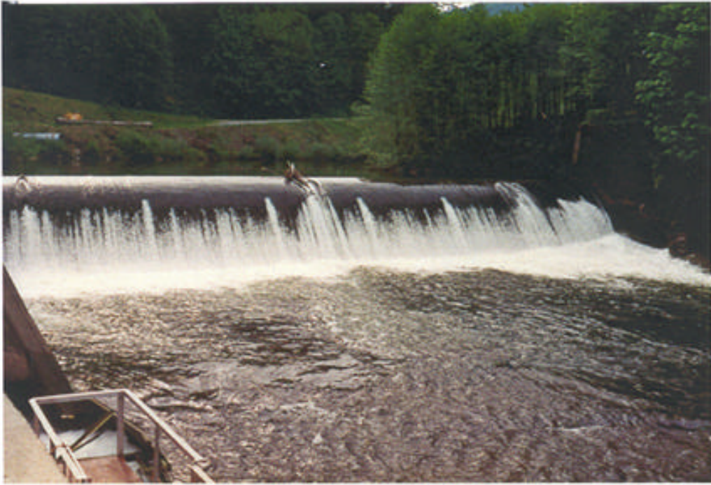
Figure Pass-5. Tacoma Headworks diversion dam, RM 61. (Source: Tacoma Public Utilities).
