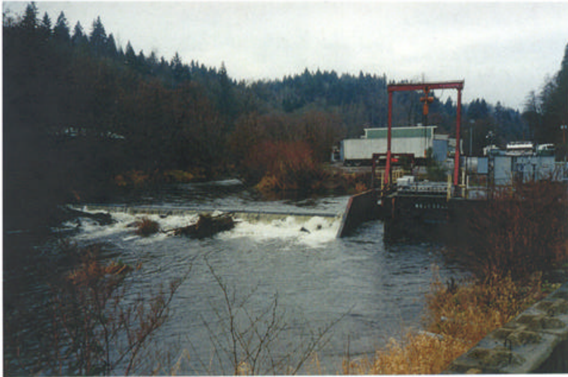
Figure Pass 15. Diversion weir and fish ladder at Soos Creek hatchery, RM 0.7, March 2, 2000 (Source R2 Resource Consultants).
