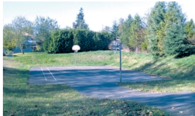
A basketball court was installed in this detention pond.
