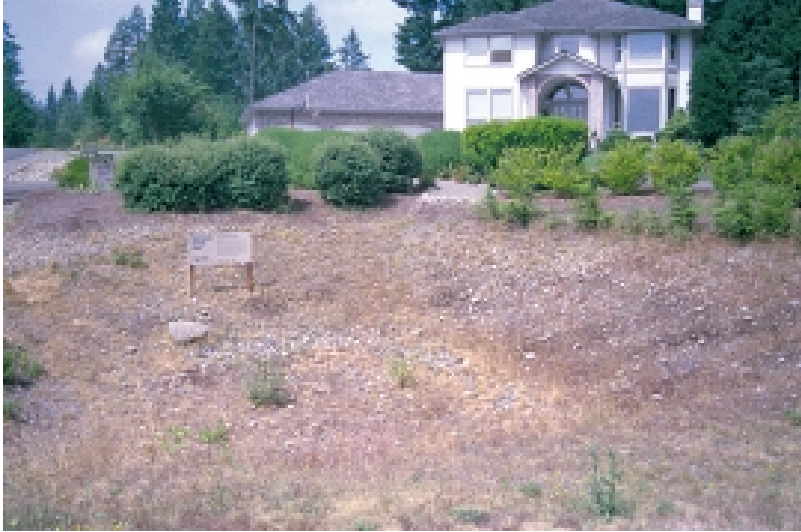
This is typical of hundreds of similar detention ponds – functional but ugly.
