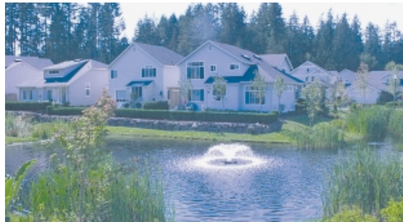
This water quality pond at Audubon Park exhibits the best in current water quality pond design – fountains, landscaping, places for people.
