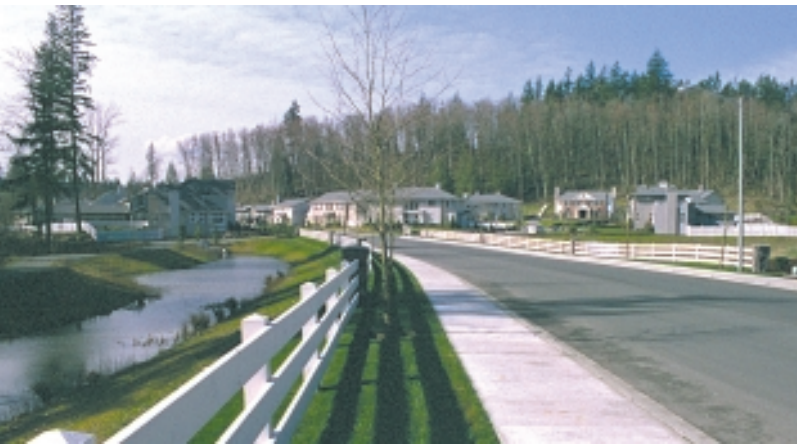
These large water quality ponds were placed on either side of the extended entry road into this community lending a pastoral and exclusive quality to the whole community.
