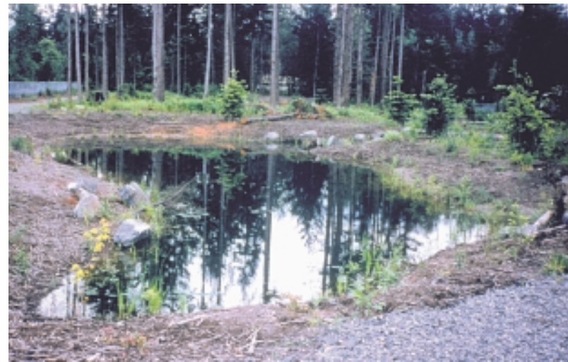
The 6th Ave. “habitat style” detention pond (case study E) uses landscape architect Peggy Gaynor’s method of spreading wood chips, planting with natives and leaving preexisting native foliage to inoculate the disturbed area.
