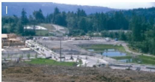
An overview of Issaquah Highlands shows how ponds are an integral part of the community.
