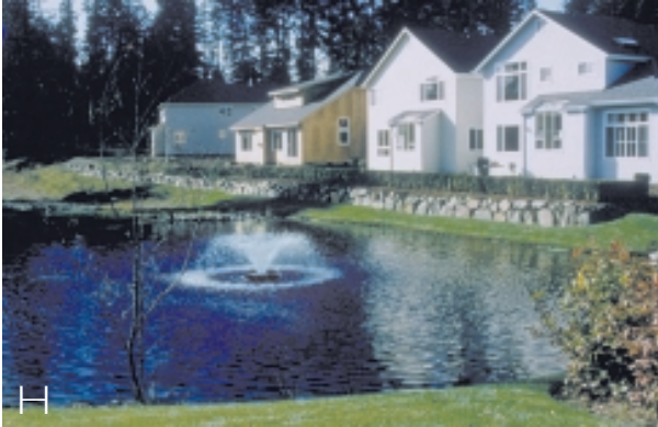
Combination water quality pond and fresh visual amenity forms the heart of Audubon Park.
