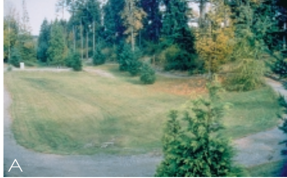
The upper end of the long detention pond/park at Evergreen shows a perimeter road.
