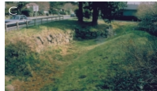
Steep rock walls provide more storage in a tight area.
