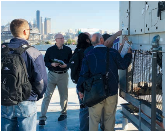
Energy Service Provider Training at King County Metro Transit Building
