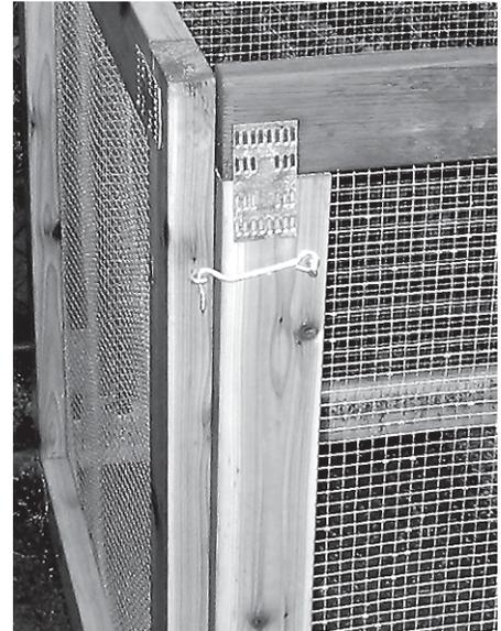
gate latches on the ends so the sections latch together.
