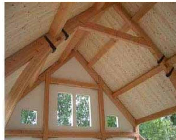
*Fig. 36* typical Bensonwood heavy timber framing
