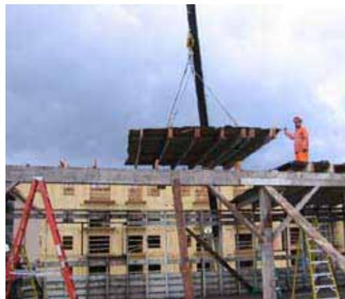
Fig. 13 panelization of roof structure
