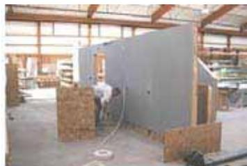
*Fig. 34* preassembly of an interior wall
