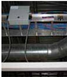
Fig. 50 electrical and telecom raceways
