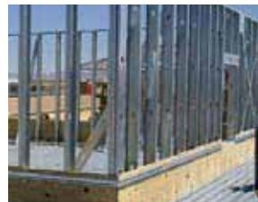
Fig. 73 light-gauge metal framing
