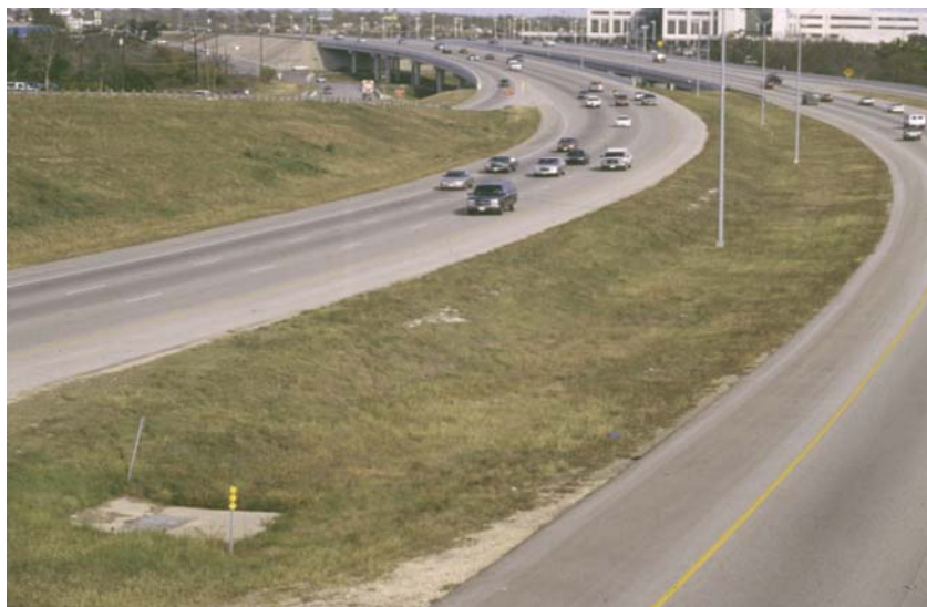
Figure 2. Median Swale Monitored in Austin, TX
