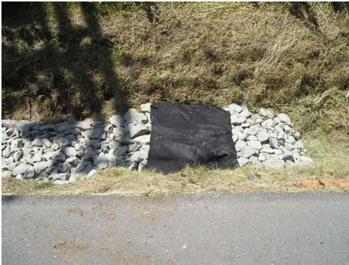
Figure 7. Treatment cell geotextile fabric filled with washed, coarse sand and wrapped.
