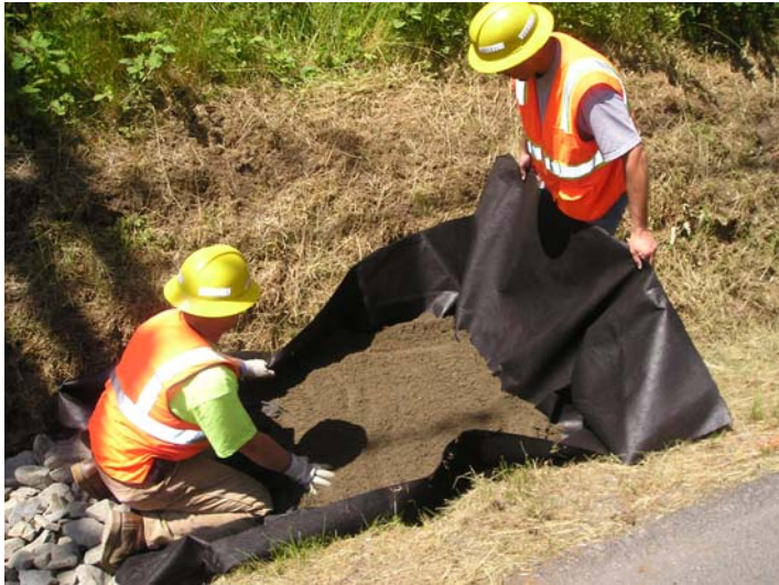
Figure 6. Crews fill the treatment cell with washed, coarse sand.
