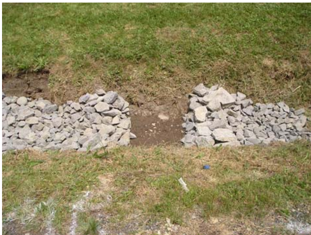
Figure 5. Lower rock ramp and upper rock ramp installation with 2-foot long gap left to allow for treatment cell installation.
