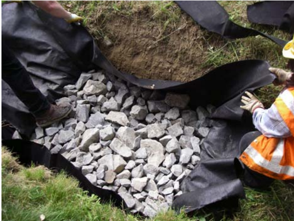
Figure 4. Splash pad trench lined with geotextile fabric, filled with angular rock mixture, and wrapped inward over the splash pad edges, which is then secured with angular rock.
