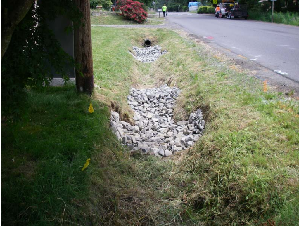
Figure 7. Completed BMPs. Lower end of ditch looking east.
