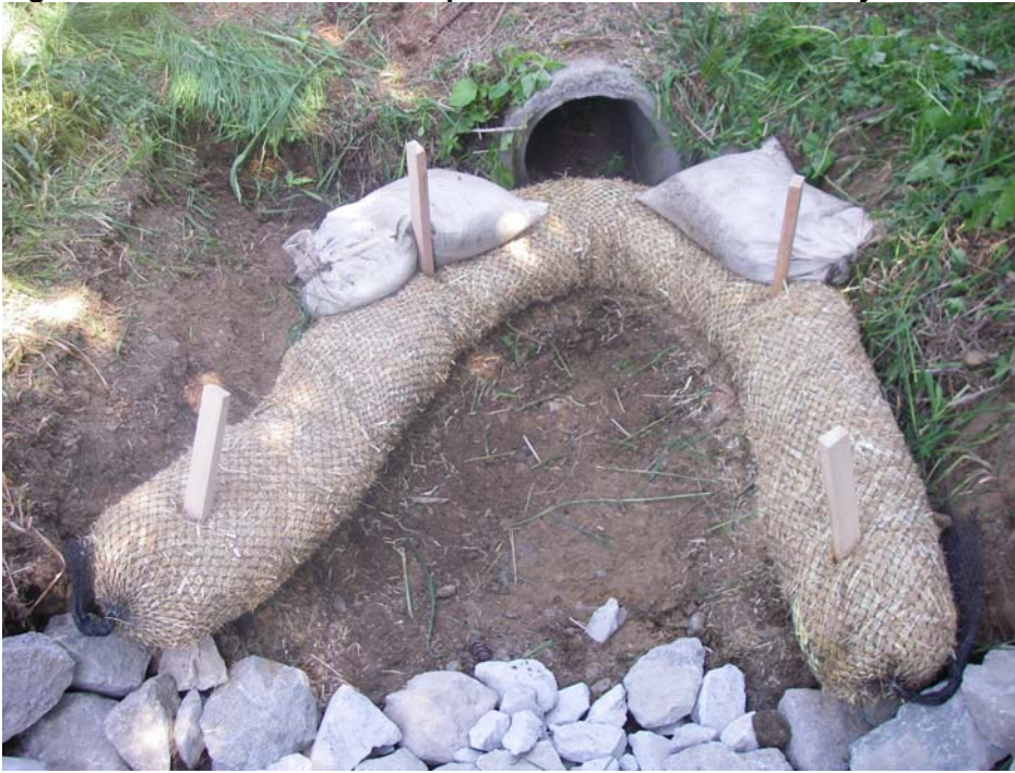
Figure 7. Straw wattle secured upstream of culvert immediately below treatment cell.
