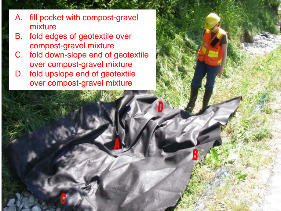
Figure 5. Compost-washed gravel mixture being placed in treatment cell.
