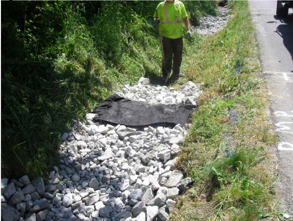
Figure 6. Compost-filled treatment cell ready for securing with rock.
