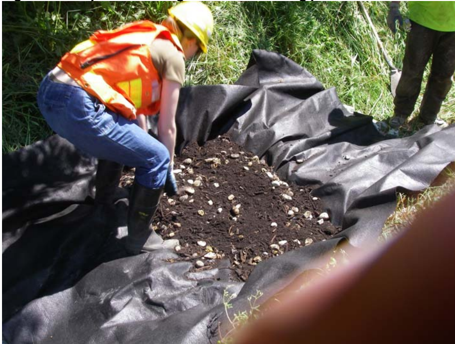
Figure 5. Compost-washed gravel mixture being placed in treatment cell.
