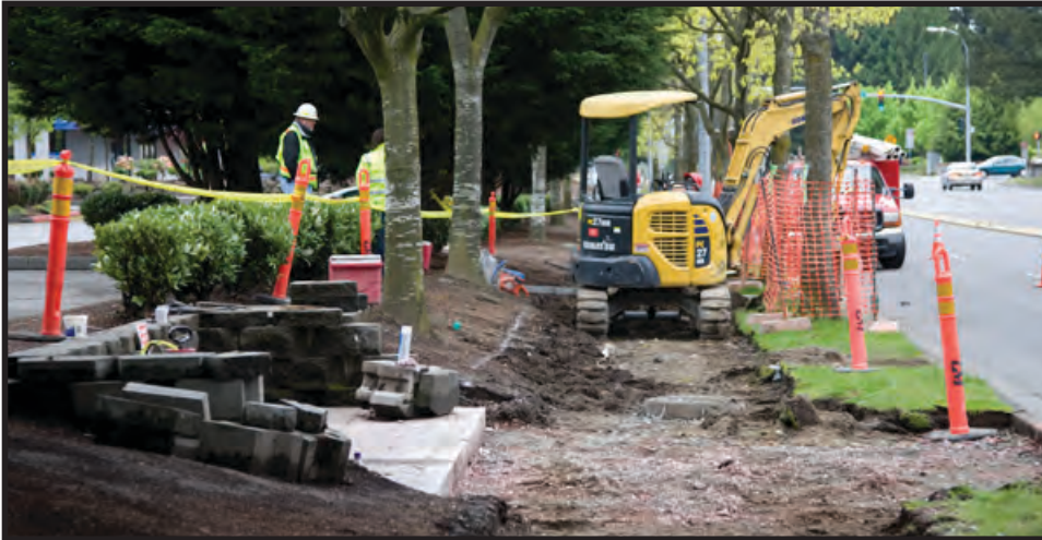
Preparations are underway for new RapidRide shelters on the Eastside.
