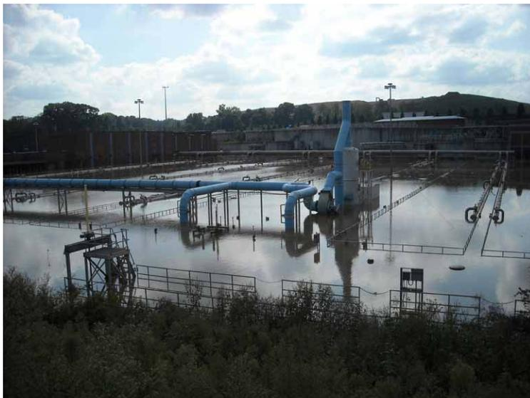
6. What were the influent concentrations for BOD, TSS, TKN, and alkalinity? Dilute wastewater was not the problem; the problem was flooding of the treatment units causing bypass of the entire plant.
