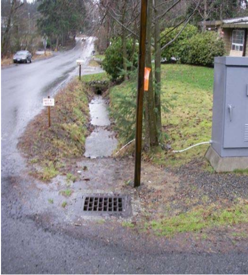
Figure 16 Stormflow Pooling above BMP Structures, SE 136 th Street
