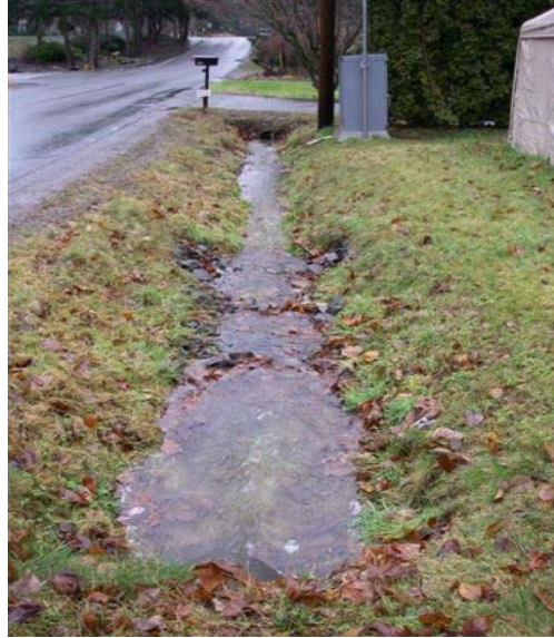
Figure 16 Stormflow Pooling above BMP Structures, SE 136 th Street
