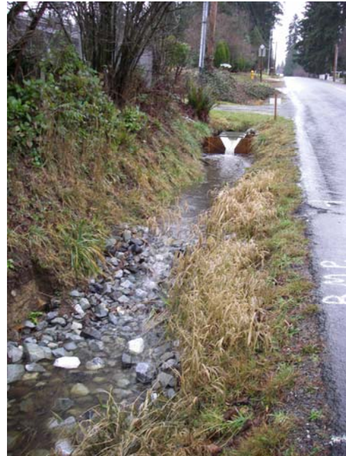
Figure 7. Stormflow Pooling above BMP Structures, 148 th Ave SE
