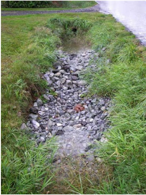
Figure 7. Stormflow Pooling above BMP Structures, 148 th Ave SE
